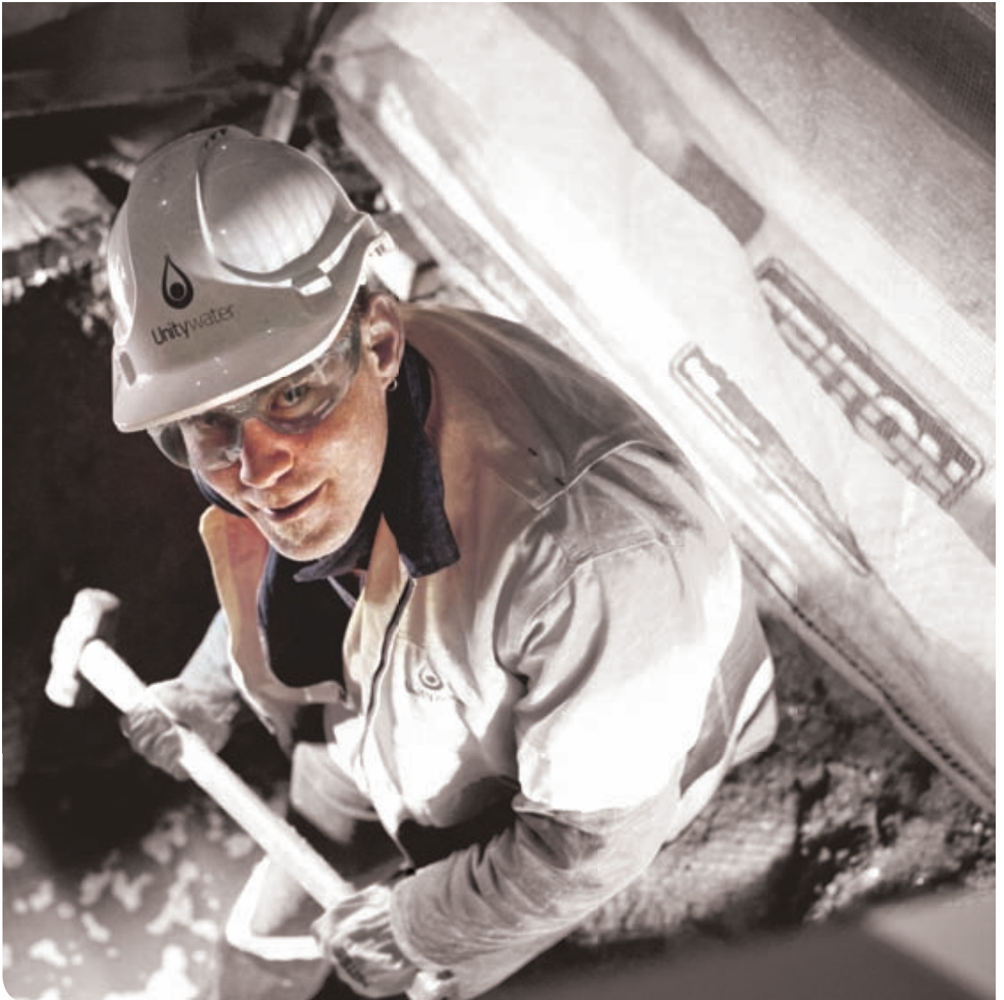
Clinton | Leading Hand Replacing Fire Hydrants — Kenilworth 11.45pm
