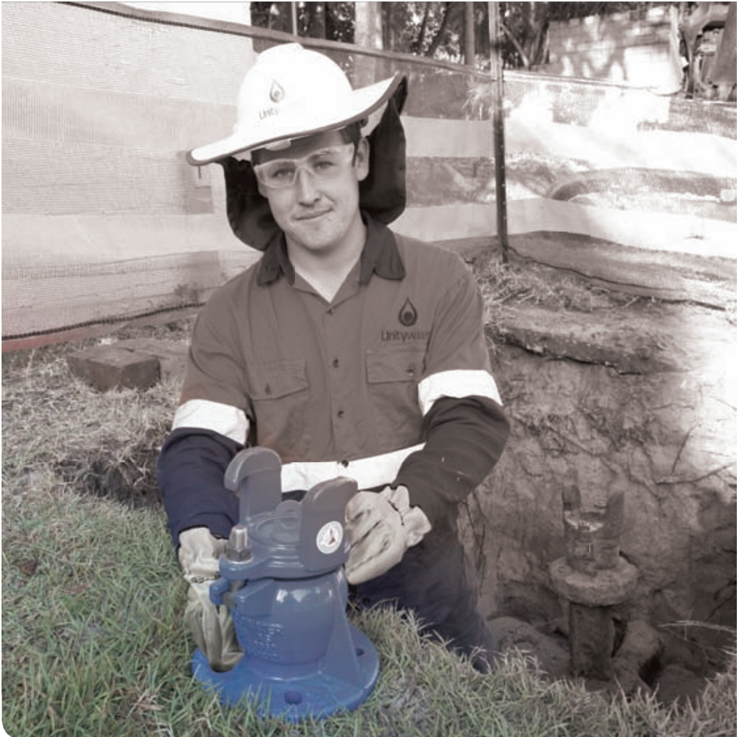
Brock | Field Worker Fire Hydrant Replacement Program — Noosa 7am
